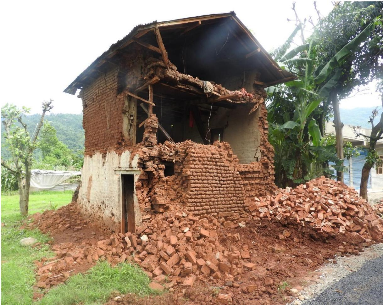
A brick-in-mud house in Bidur Municipality, Nuwakot that suffered damage during the earthquake.
